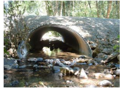
Replaced Culvert in Mohawk Watershed
