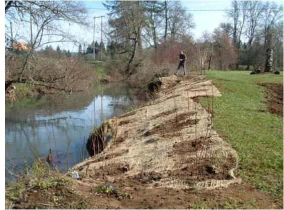
Bank stabilization project
