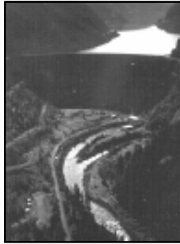
The 1998 water quality report includes recommendations for temperature control devices to be installed at Cougar Dam.
