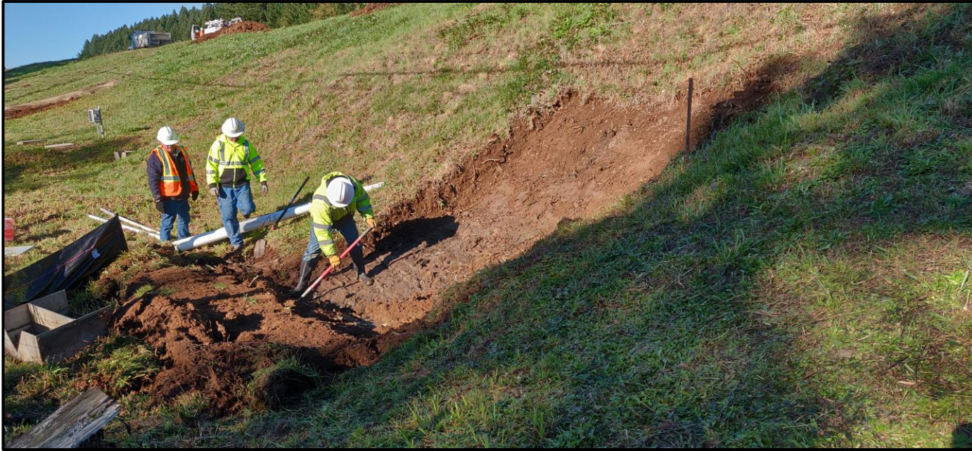
Sediment filter and weir installation in the Cogswell Reach
